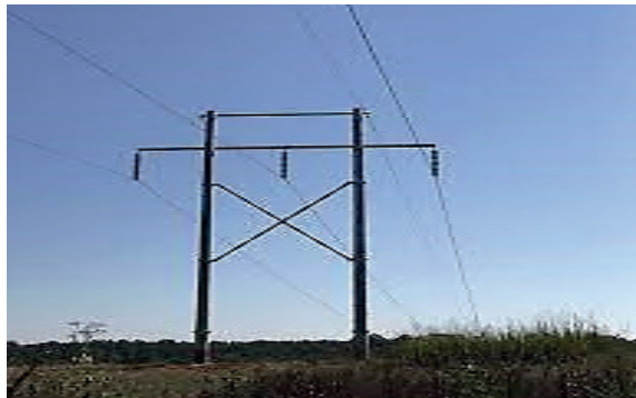
Fig 2.19: Medium Voltage Transmission Line
