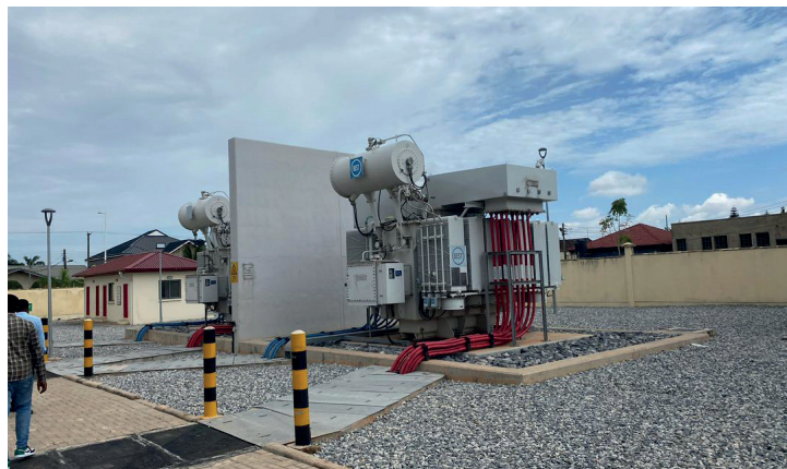
Fig 2.27: Power Transformer in a Substation
