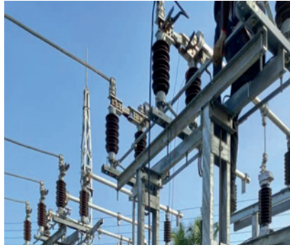
Fig 2.26: Circuit Breakers and Disconnect Switches
