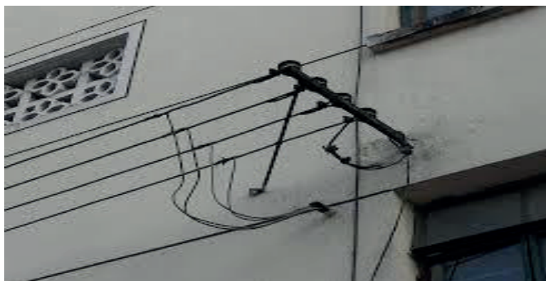
Fig 2.35: Three-phase line connected to a House
