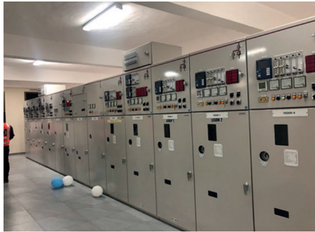
Fig 2.32: Monitoring and Control Panel of a Power Distribution Substation (Source: ECG Station)
