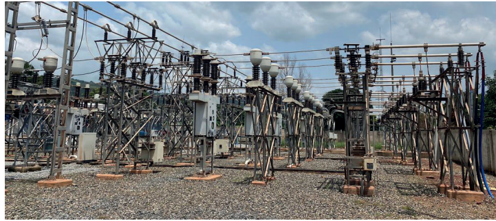
Fig 2.29: Switchgear in a Substation (Source: ECG Substation)
