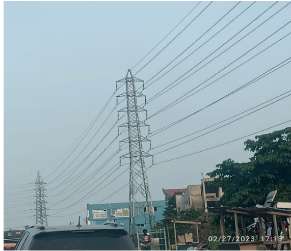
Fig 2.18: High-voltage Transmission Line (33 kV)
