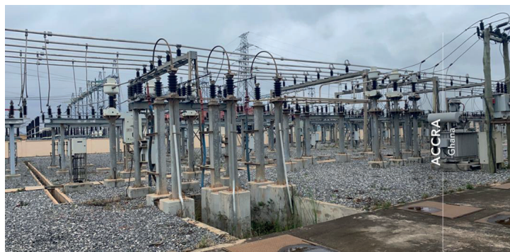
Fig 2.28: Busbars in a Substation
